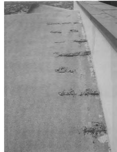
Concrete deterioration and corrosion of embedded reinforcing steel on 10 foot-wide, high roof “overhang”. Note absence of deck coating or waterproofing system on exposed horizontal concrete surface.
