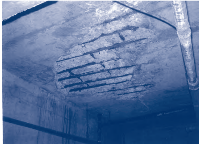
Corrosion of reinforcing steel and concrete deterioration of upper level Parking Garage ceiling due to long-term water intrusion, requiring wholesale demolition of 12 inch-thick concrete slab.
